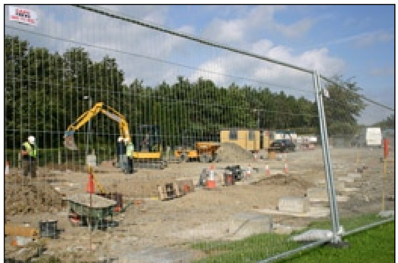
Construction of a new sixth form centre.
