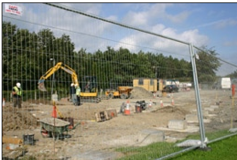
Construction of a new sixth form centre.
